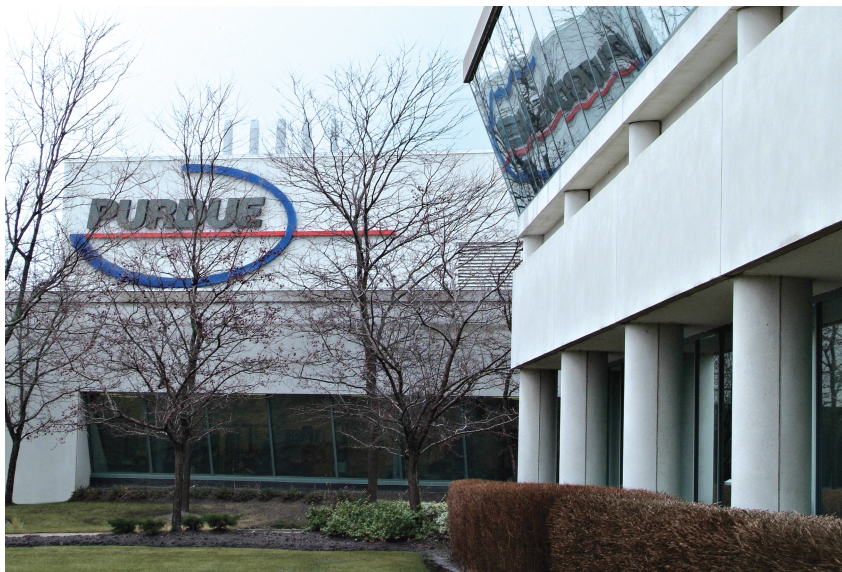
Located in Pickering, Ontario, Purdue's impressive Canadian facility houses administration, research, manufacturing and sales support functions.
